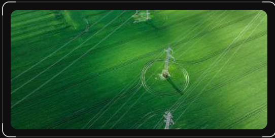
— AERIAL VIEW OF ELECTRIC TOWERS IN GREEN FIELDS
