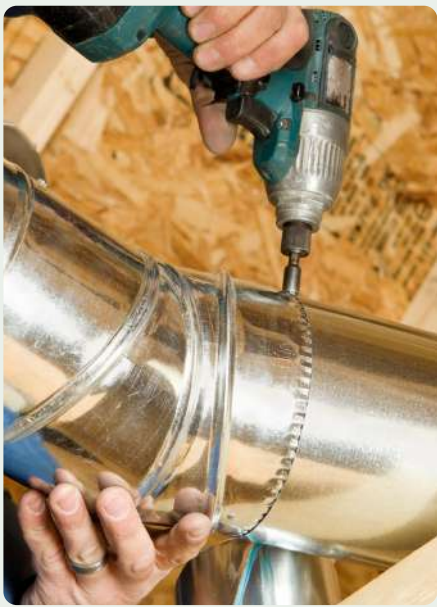
-- A WORKER INSTALLING A VENT DUCT
