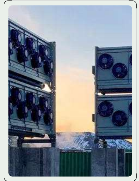
— CLIMEWORKS' DAC+S FACILITY "ORCA" IN ICELAND
