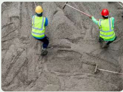
-- WORKERS MIXING CEMENT
