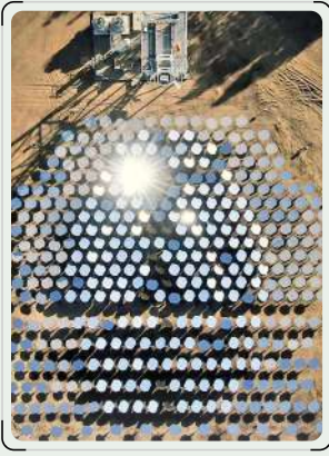
STARTUP HELIOGEN USES FIELDS OF AI-CONTROLLED MIRRORS TO HARNESS THE POWER OF THE SUN.
