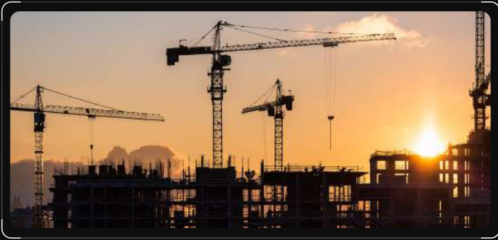
-- A CONSTRUCTION SITE AT SUNSET
